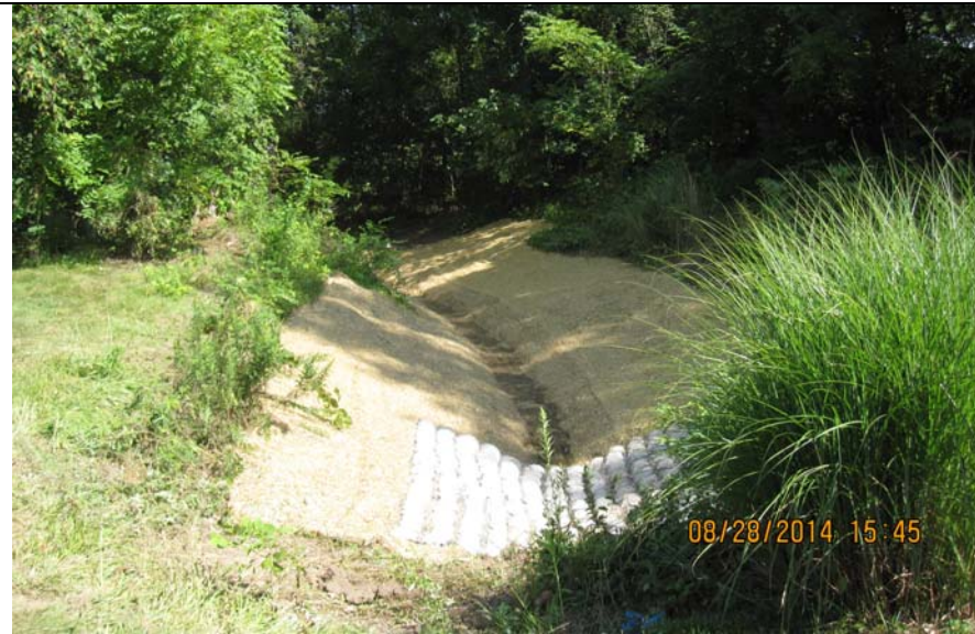
Photo #1: Placed straw matting and flex-a-mat within the finished ditch grades.
