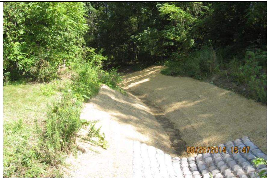
Photo #4: Placed straw matting and flex-a-mat within the finished ditch grades.
