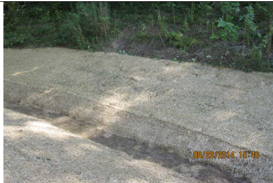
Photo #3: Placed straw matting within the finished ditch grades.
