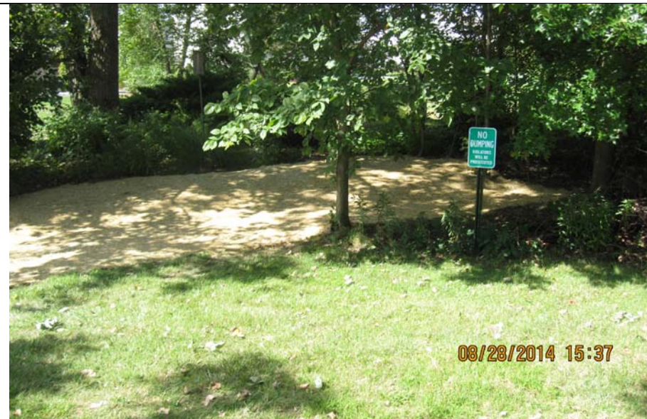
Photo #3: Placed straw matting within the finished grades.
