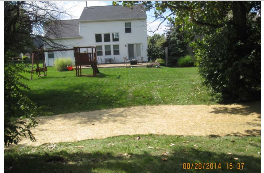
Photo #2: Placed straw matting within the finished grades.
